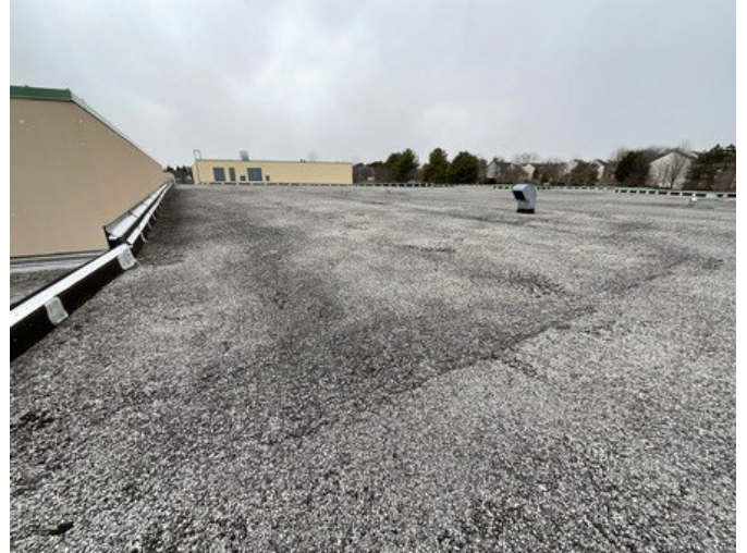
14 - MODIFIED BITUMEN ROOF
