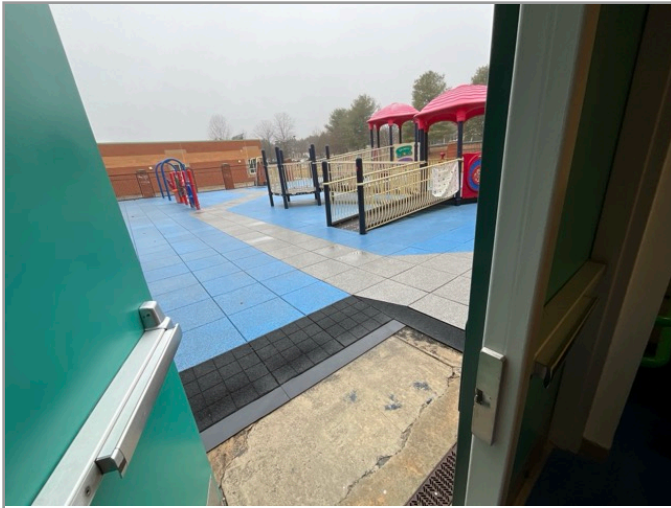
ACCESSIBLE ROUTE TO PLAYGROUND
